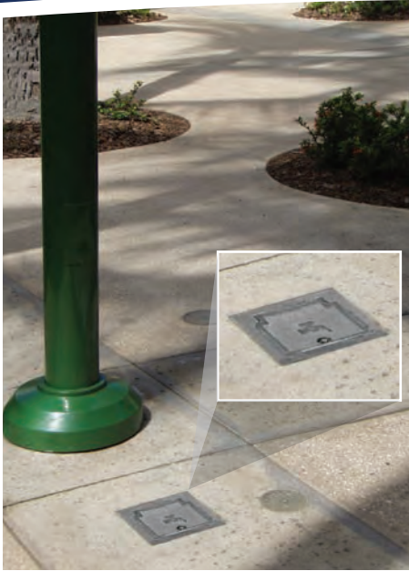
Boxed Ground Hydrant
